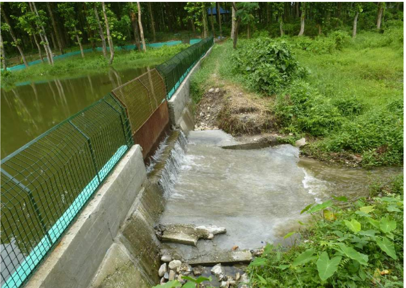
New inlet (above) and outlet of TRCC lake with new fencing around whole lake
